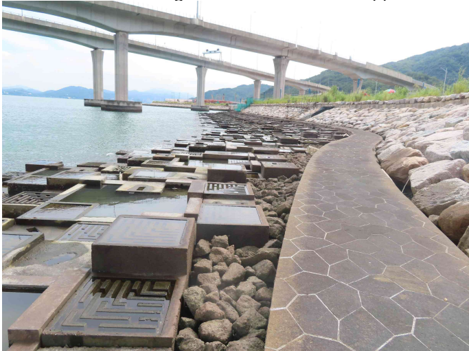
General View of Rocky Eco-shoreline
