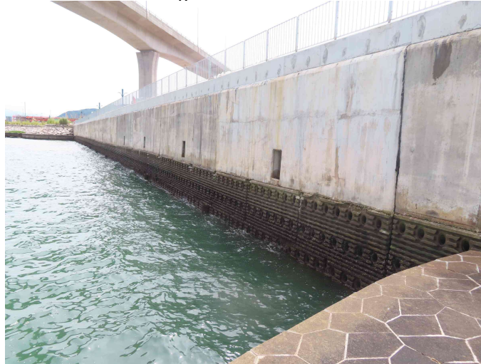
General View of Vertical Eco-shoreline
