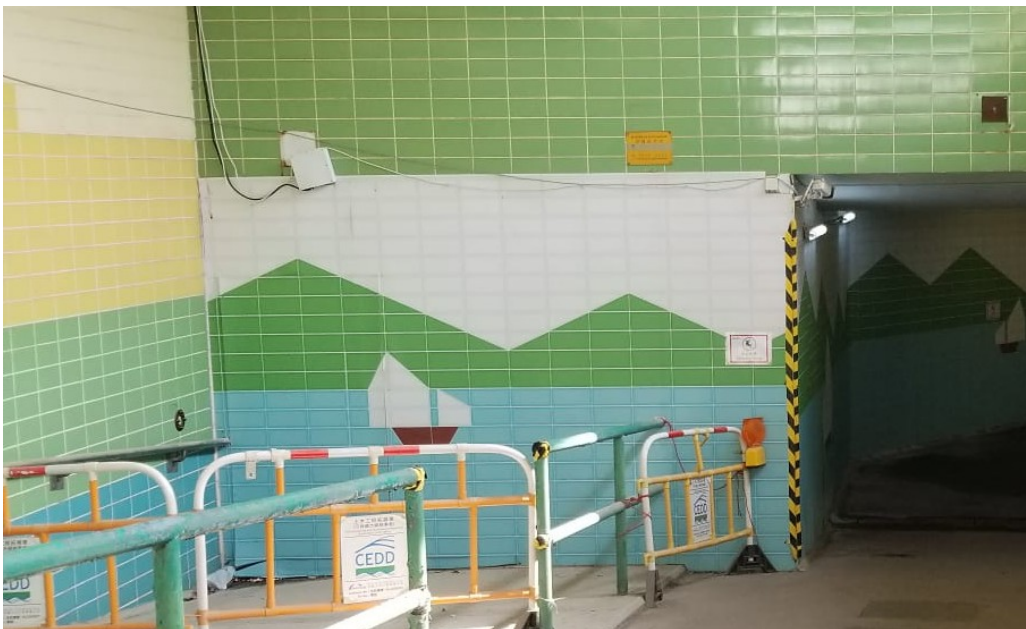
Photo 3 – Erection of site hoardings in unobtrusive colours
